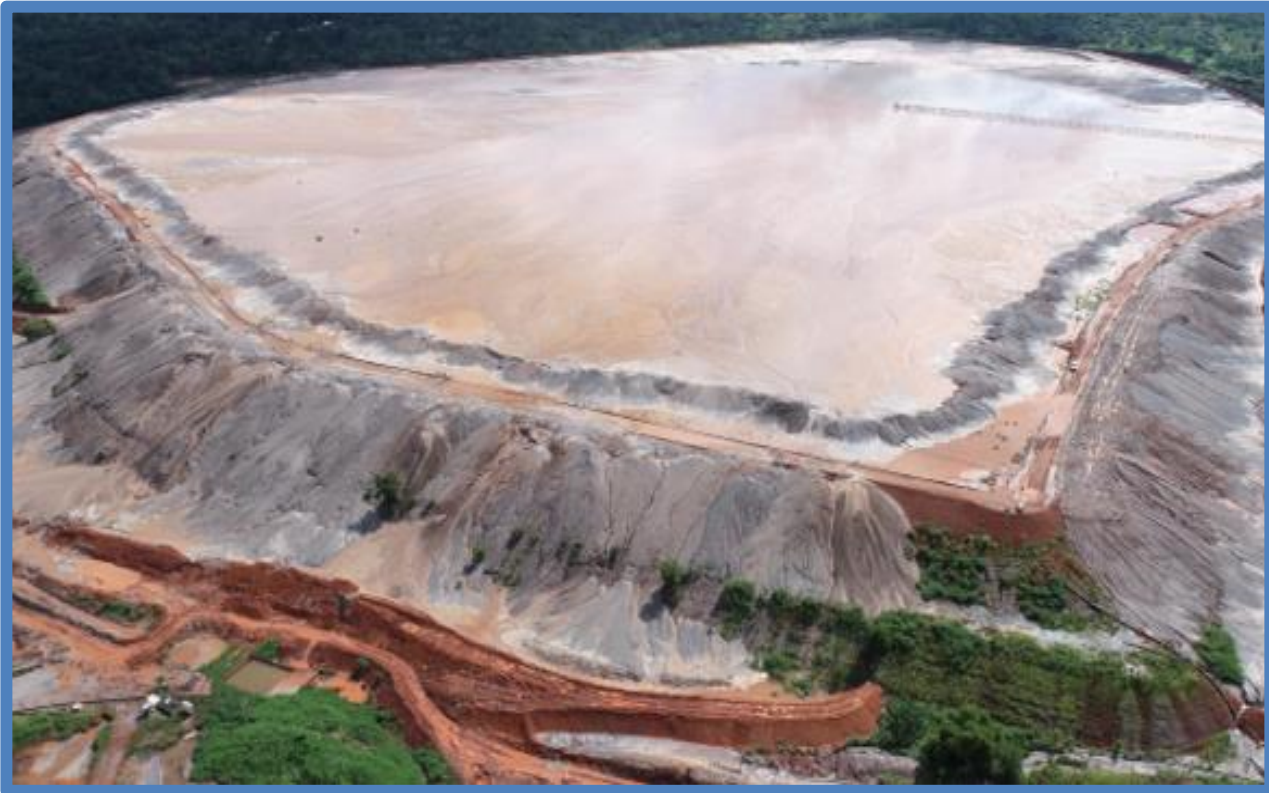
Figure 2- 16: Overview of Valley B TSF – Current View of Cyclone Deposition
