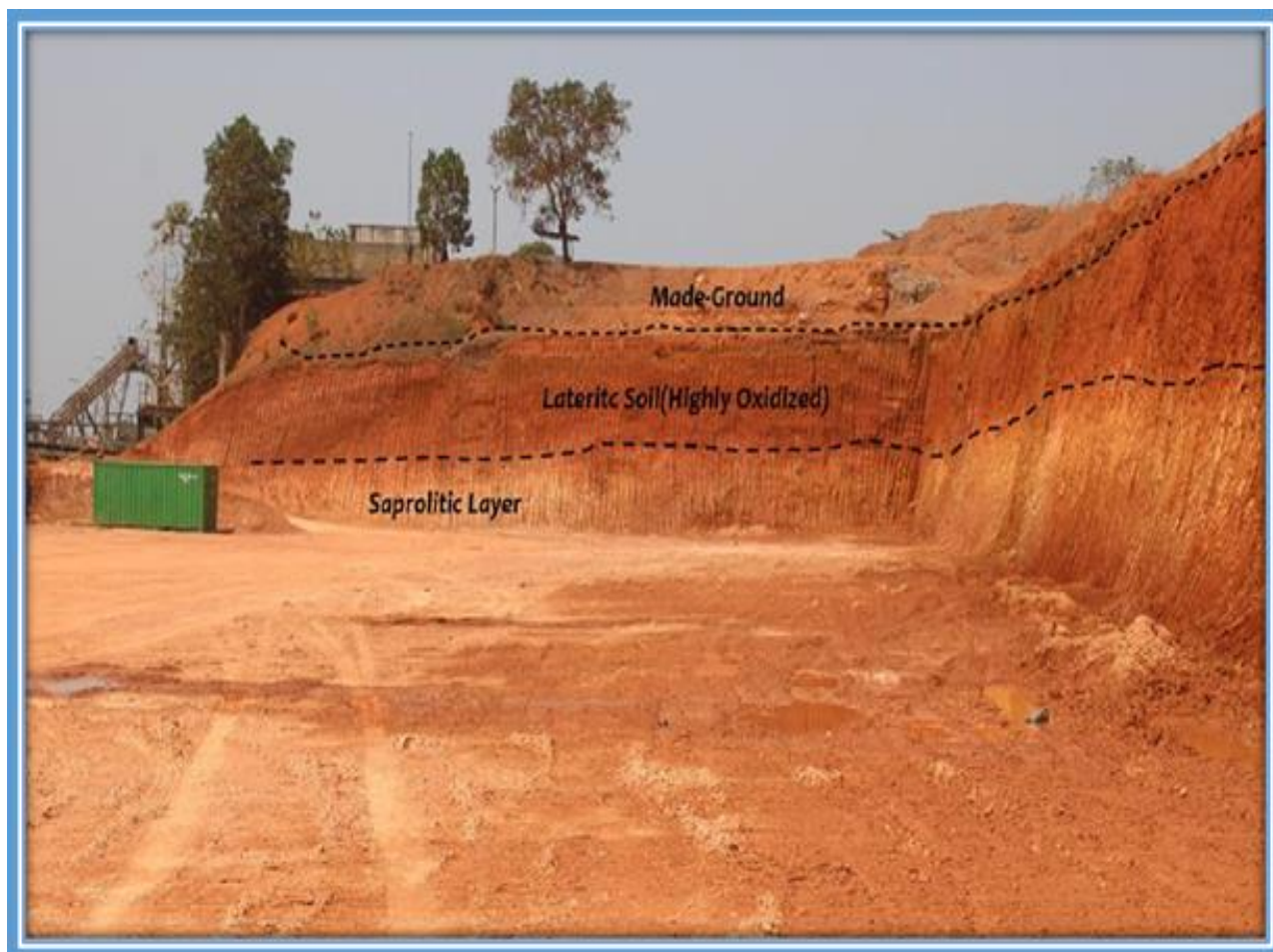
Figure 4- 12: An Exposed Face of a Newly Excavated Area Where the New Power Plant is to be Built.
